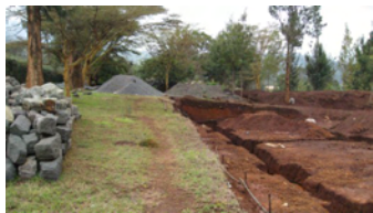
Digging the hospice foundations at Kijabe
